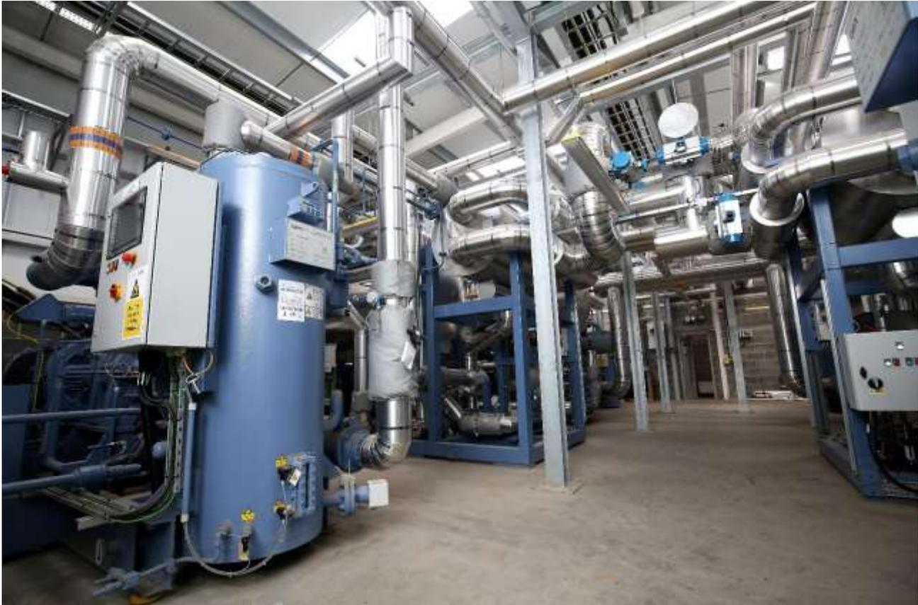
**Photo 2, caption:** The use of ammonia heat pumps in the Gateshead project is a reflection of the advancement in the development of district heating. (Photo: GEA)
