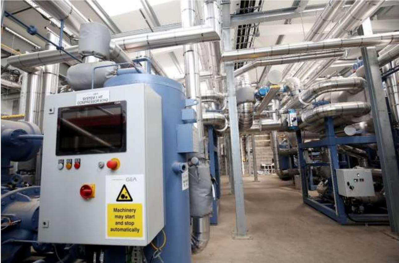
**Photo 1, caption:** GEA is at the forefront of technology solutions for tackling climate change and supplying district heating projects like this one in the Northeast of England. GEA heat pumps are at the center of the Gateshead Mine Water Scheme, the largest mine water heat recovery scheme of its kind in the country. (Photo: GEA)
